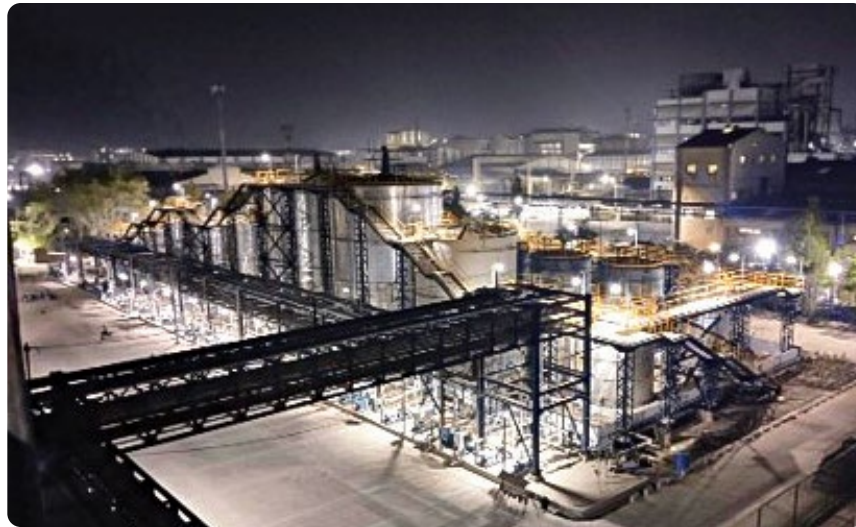
Night view of our Ankleshwar plant
