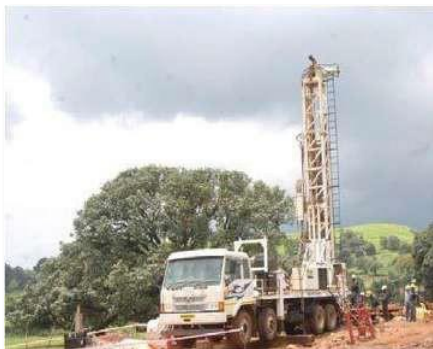
CBM Exploratory Drilling at Satpura, MP for Dart Energy
