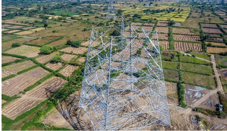
Tower erection work
