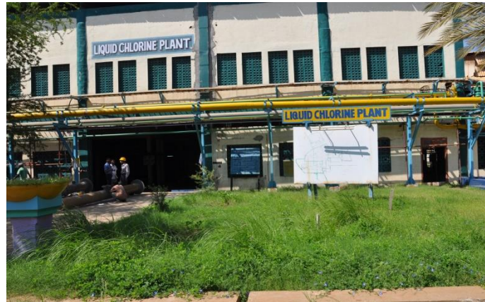
Liquid Chlorine Plant
