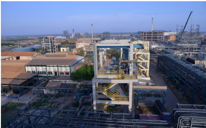
Hydrochloric Acid Plant
