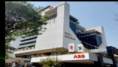
B&R Industrial Automation, Pune*
