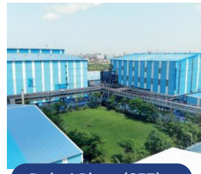
Dahej Plant (SEZ)
