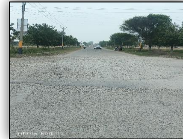
Road patch work for safe passage
