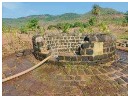
Repairs of Water Wells, At- Nivi Adivasiwadi , Roha Raigad
