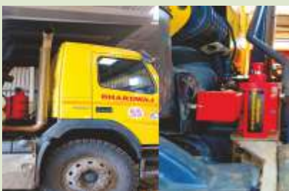
Automatic Fire Detection and Suppression System
