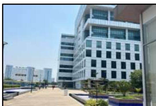
View of Tower G3 and C2
