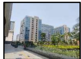
Amenity Block 2 of Subject Property
