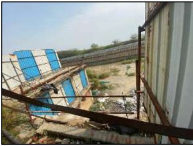
View of Block 4A & 4B (Future Development)
