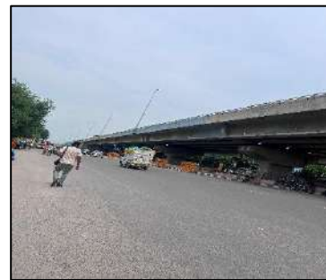
View of NH -48 (Secondary access road)
