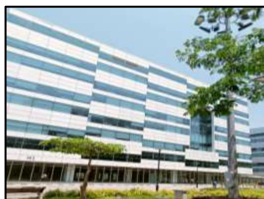
View of Tower G1
