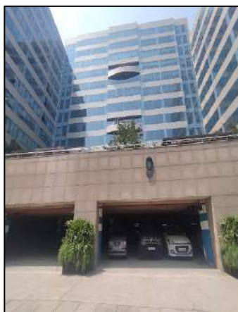
View of Tower 9
