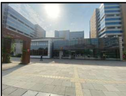
View of Amenity Block (Block 7)
