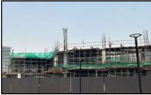
Under-Construction Commercial Block
