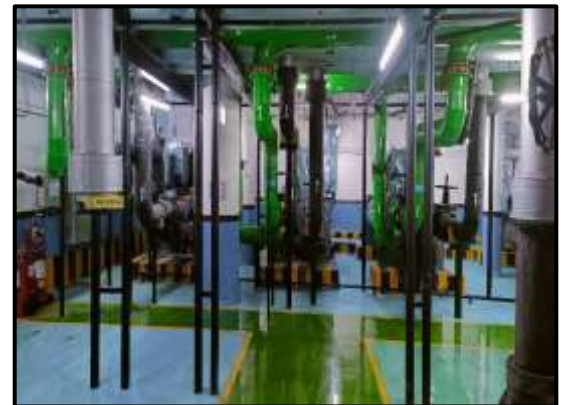
View of Generator Room
