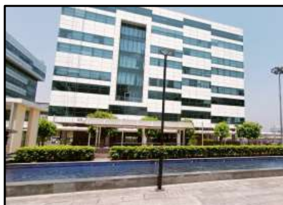
View of Tower G3
