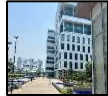
Tower G3 & C2 of Subject Property
