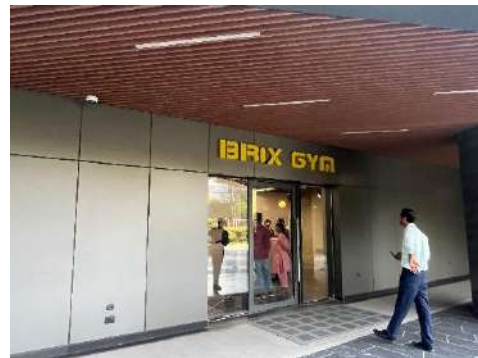
Internal View of Subject Property
