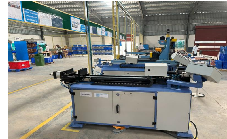
Unit 5 Copper Tubing Section
