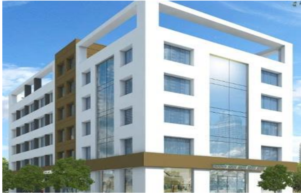
Unit 1 EMS and LED Lighting 48,000 sqft. Satpur, Nashik
