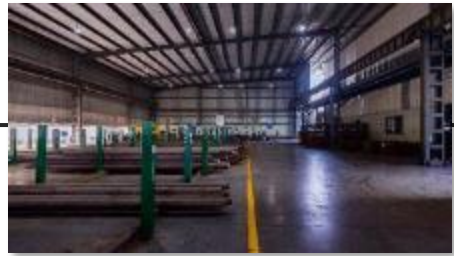
Covered Raw Material Yard
