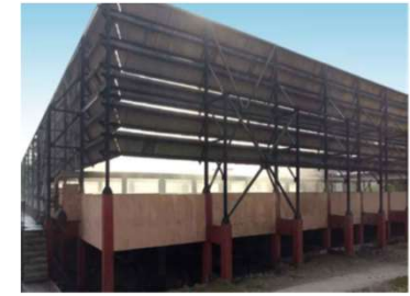
Mist Cooling System
