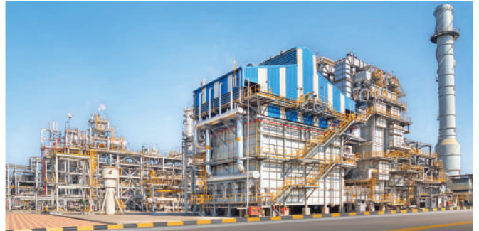
Ammonia Process Plant – Reformer Area
