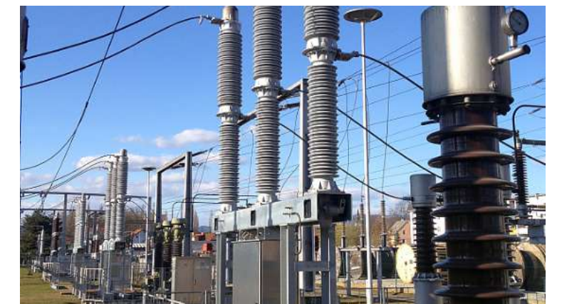
8. Instrumental Transformers
