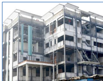
Commercial building, Delhi
