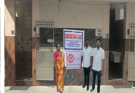
Toilet for school children in village
