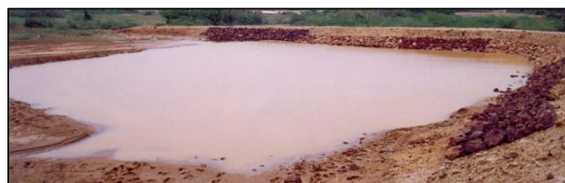
Construction of Nala Plugs
