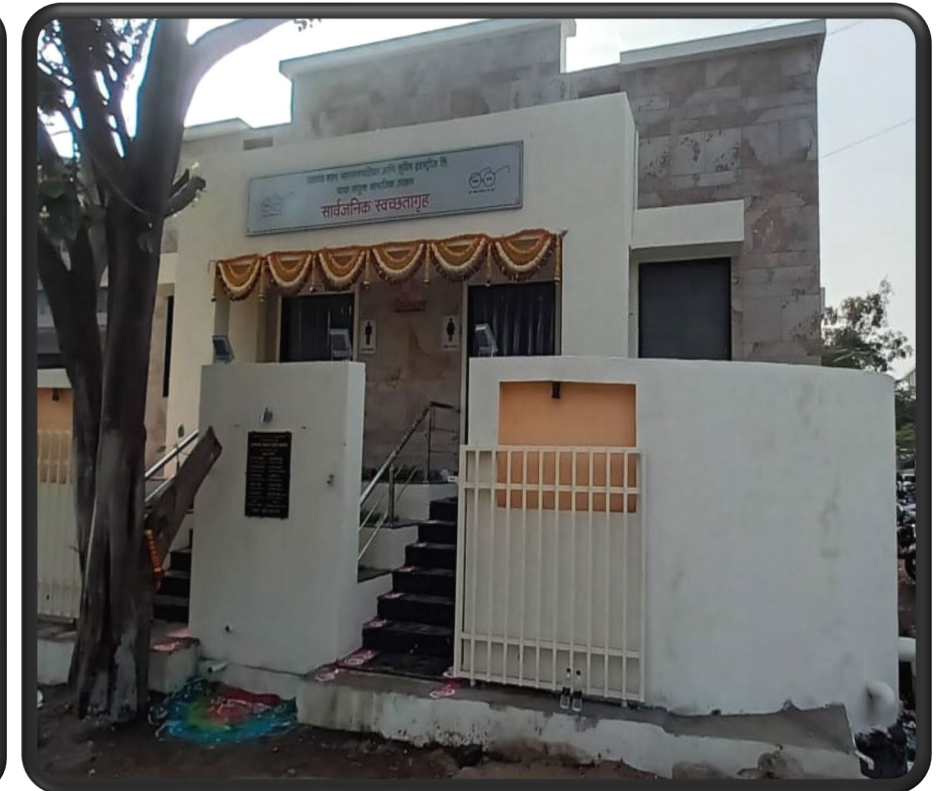
Public Sanitation Facility at Jalgaon (Maharashtra)
