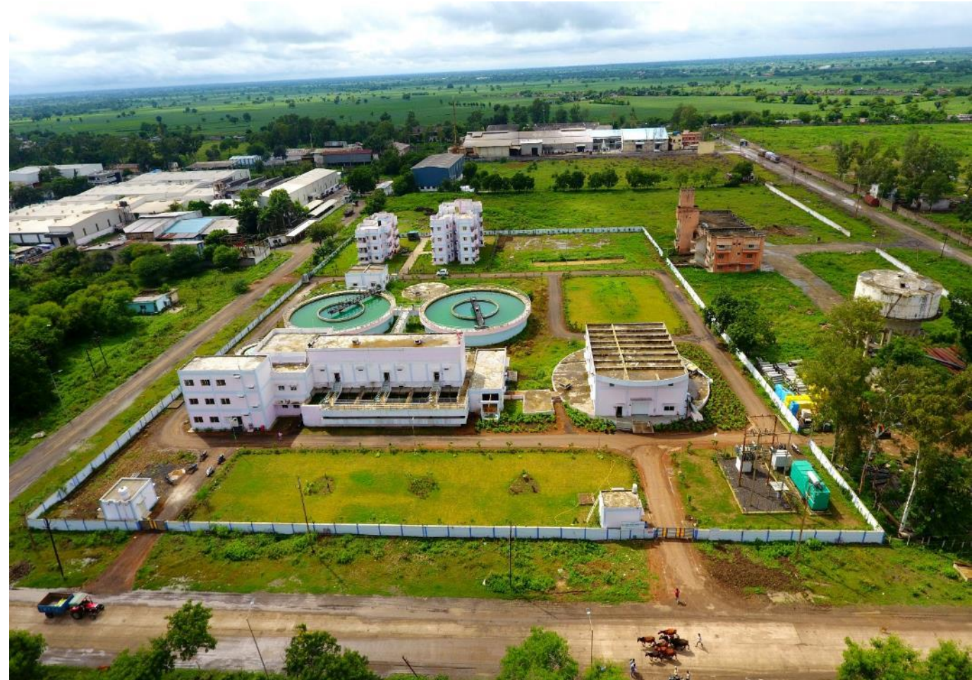
Industrial Water Treatment Plant, Dewas, Madhya Pradesh
