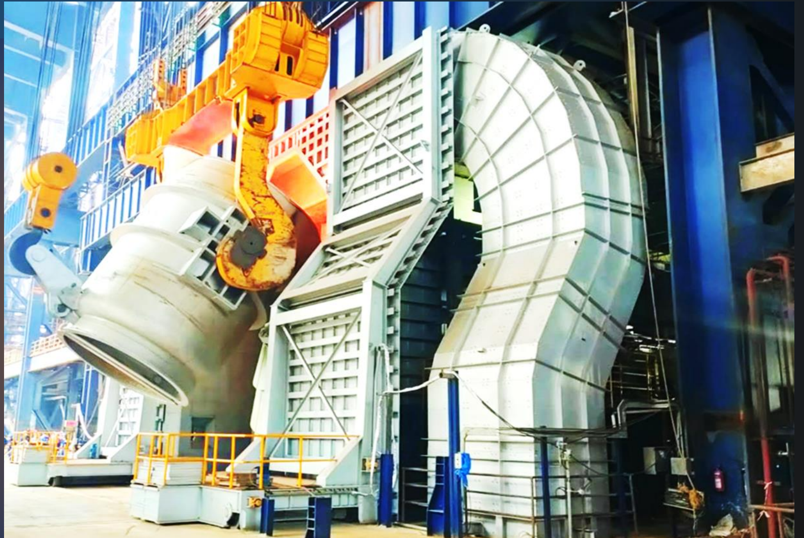
Steel Melting Shop for a reputed client in Maharashtra
