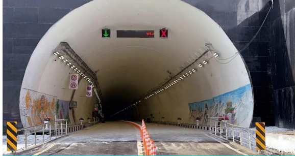
Sela Tunnel, Arunachal Pradesh
