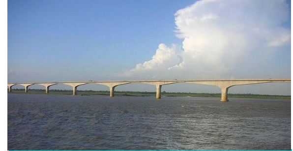
2 Lane Bridge over river Brahmaputra, Assam
