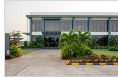
Laid foundation for Oncology OSD Plant in Visakhapatnam
