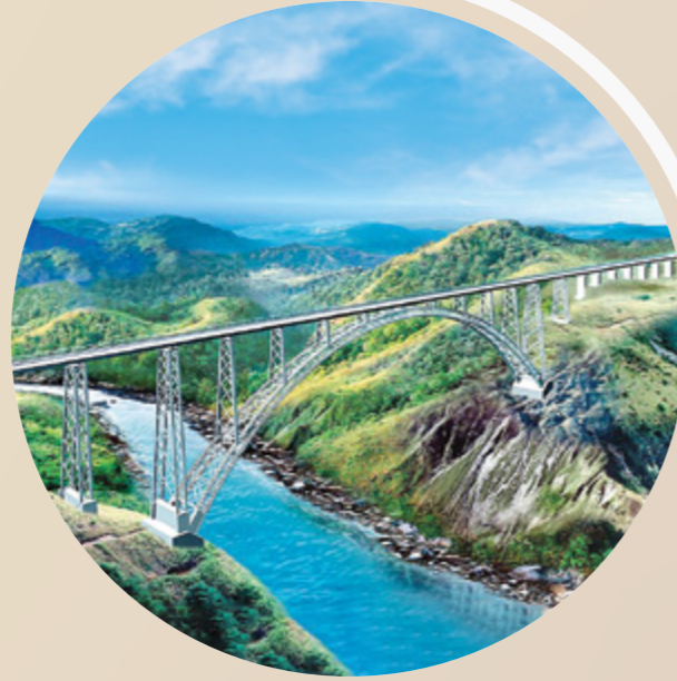
The Chenab Rail Bridge
