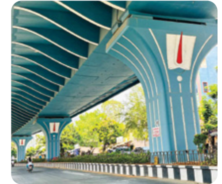
Srinivasa Sethu Flyover Project, Tirupati
