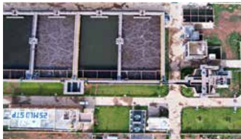
25 MLD STP, Jagdalpur, Chattisgarh
