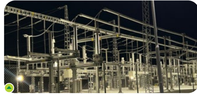
Substation Works in Sweden
