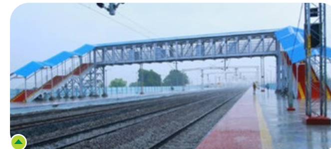
Umdanagar Mahabubnagar Doubling Project
