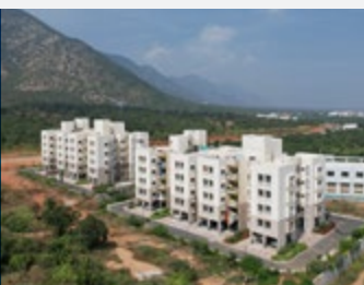
Secured First International Building Project
