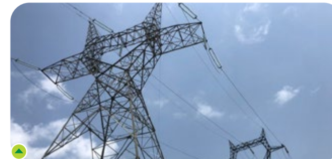
225 kV Single Circuit line in Cameroon
