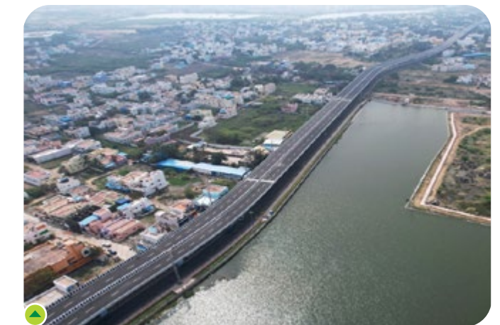
Madurai Chettikulam Flyover, Madurai
