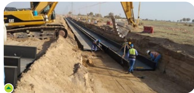
Underground cabling works in Dubai
