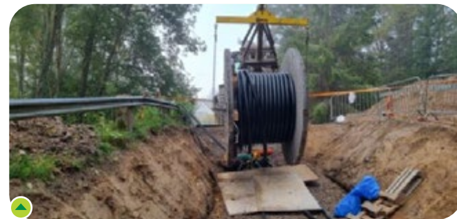
Underground cabling works in Sweden
