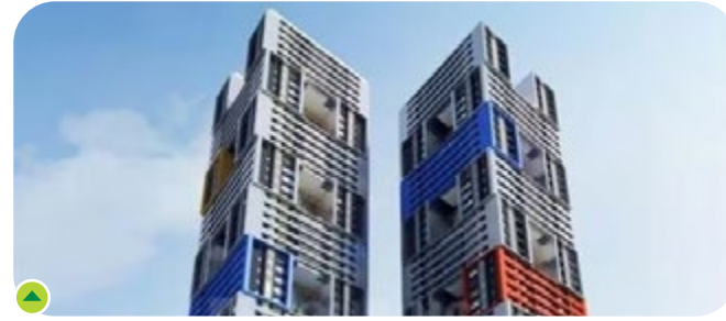
Adhiraj Samyama Township (58 storied towers - tallest in Navi Mumbai)
