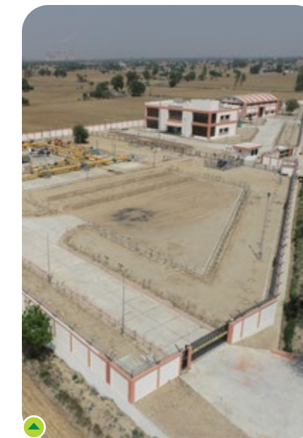
Mallavaram-Bhopal-Bhilwara-Vijaipur RFCL Connectivity Pipeline Project
