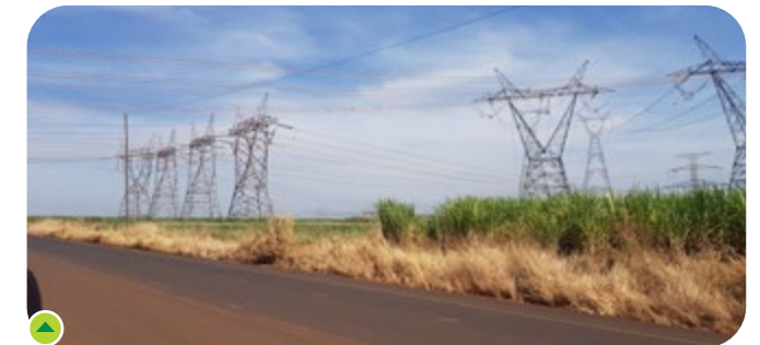
500 kV Double Circuit line in Brazil
