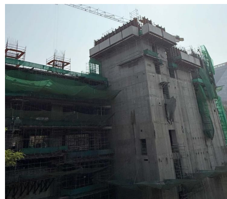
Yerwada, Pune (0.9 msf) Under Construction
