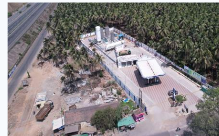
LNG/LCNG fuel stations
