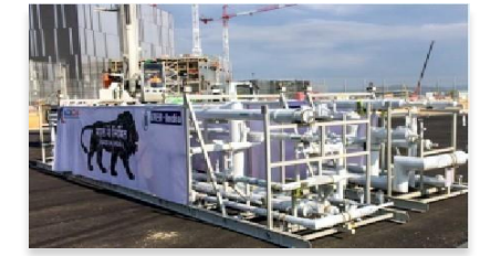
Multi-core Cryoline Warmlines
