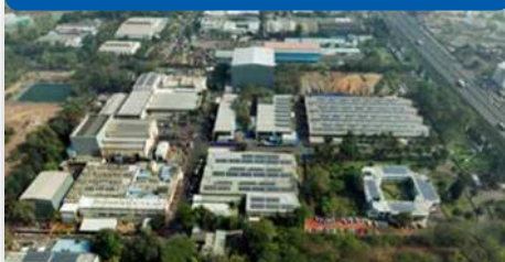
Switchgear manufacturing unit Nashik, Maharashtra
