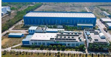
Motors & Drives manufacturing unit Bhopal, Madhya Pradesh
