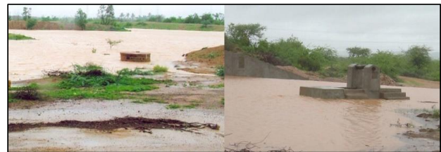
Recharging Check dams, Storage Tanks
