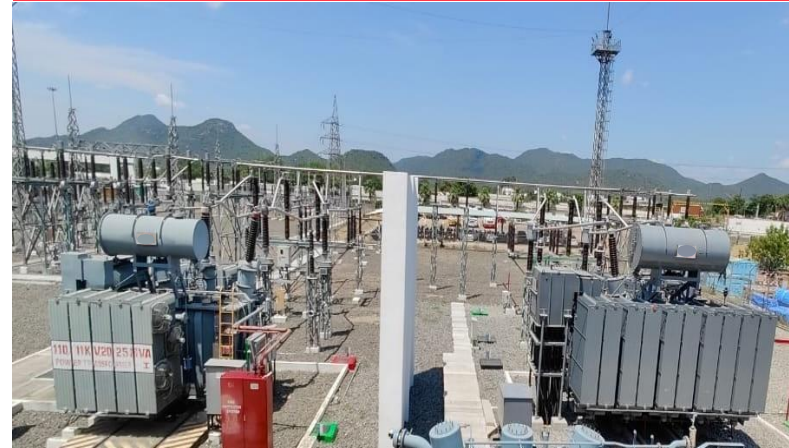
110kV/11kV AIS 1X12.5MVA 2X62.5MVA Trafo Bay Extn for industries, Trichy
