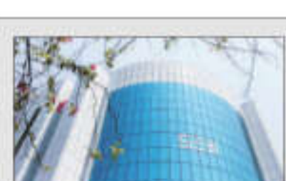
■ Shareholders of exchanges can directly hold the entire equity, who can then be free to trade their shares in clearing corporations
