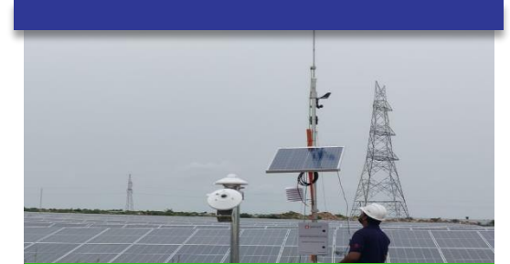
295.68 MWp Ground Mounted project at Kurnool, Andhra Pradesh
