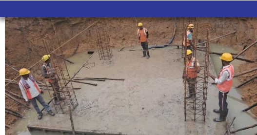
78 MWp Ground Mounted project at Tamnar, Chhattisgarh
