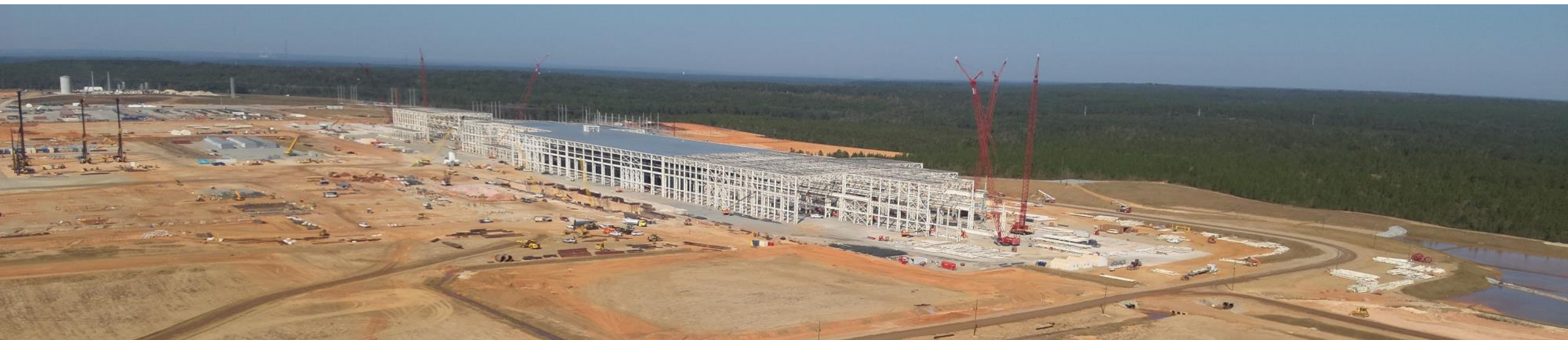
Bay Minette site and construction, October 24, 2024
