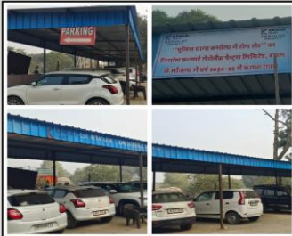
Construction of Tin shed for Kasola Thana Vehicle Parking
