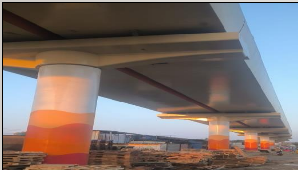
Mumbai Metro line 5 Thane Bridge Project
