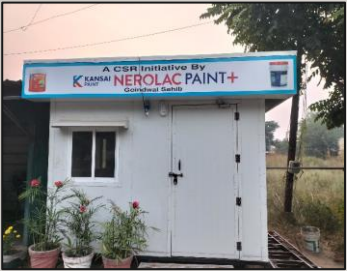
Security Post (Portable Cabin) at Urban Estate, Kapurthala
