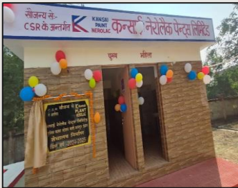
Construction of Toilets at Jainpur Fire Station, Jainpur
