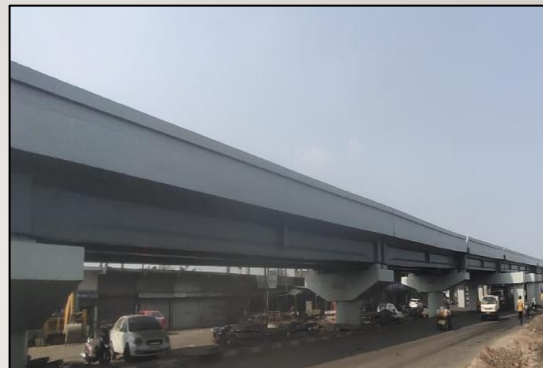
MRIDC Bridge Project (Chandrapur)
