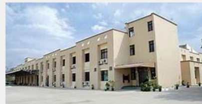
Eicher Engineering Component – Dewas
