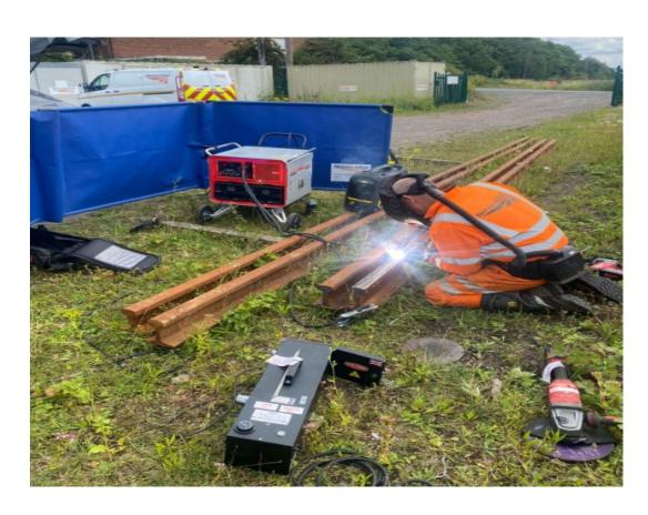
THIS BATTERY POWERED WELDING MACHINE IS BEING USED ALONG WITH ARC SENSING MIG/ MAG WIRE FEEDER IN EUROPE FOR RAILWAY TRACK MAINTENANCE
