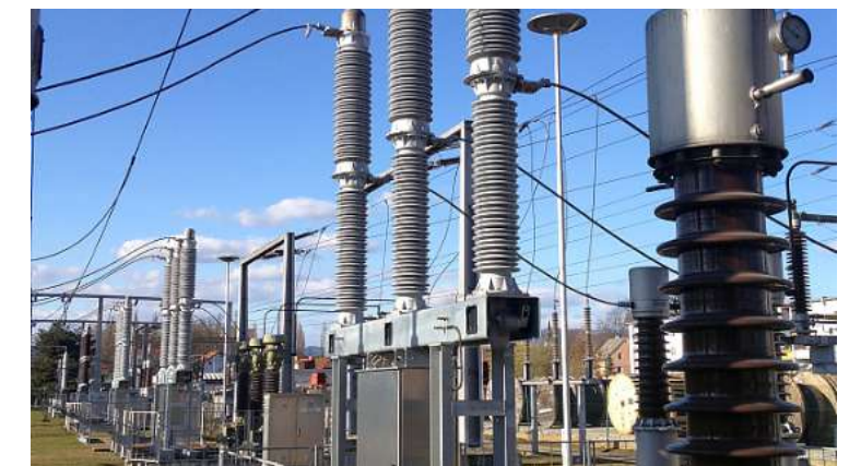
8. Instrumental Transformers
