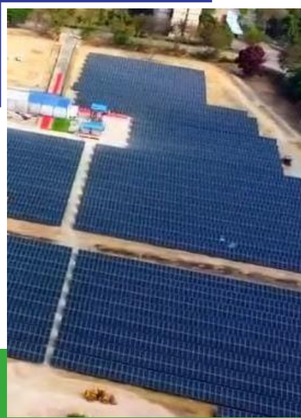
6.5MWp Ground Mounted Project at Raigarh, Chhattisgarh
