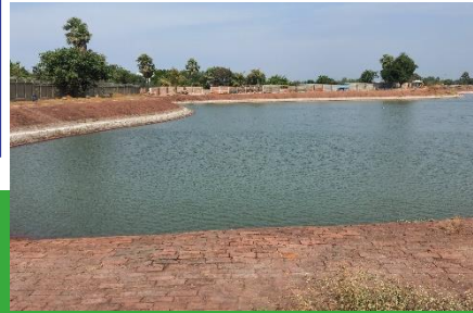
1.090 MWp Floating Solar power project at Gujarat
