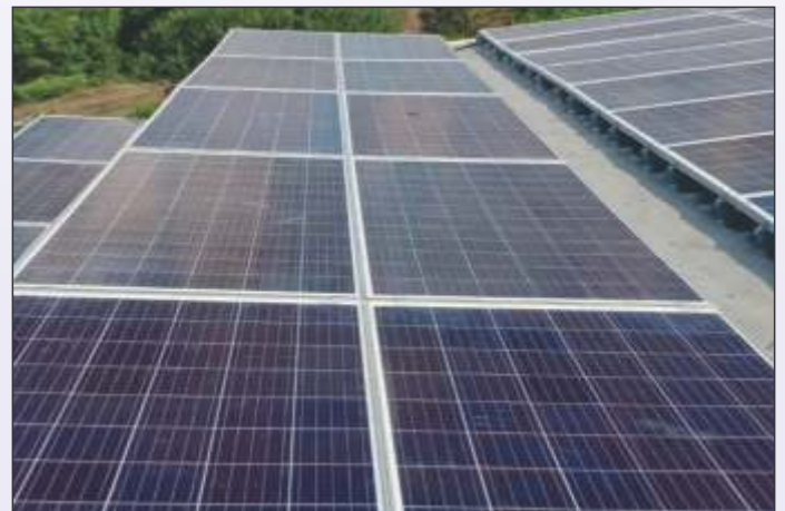
Installation of Solar Panels
