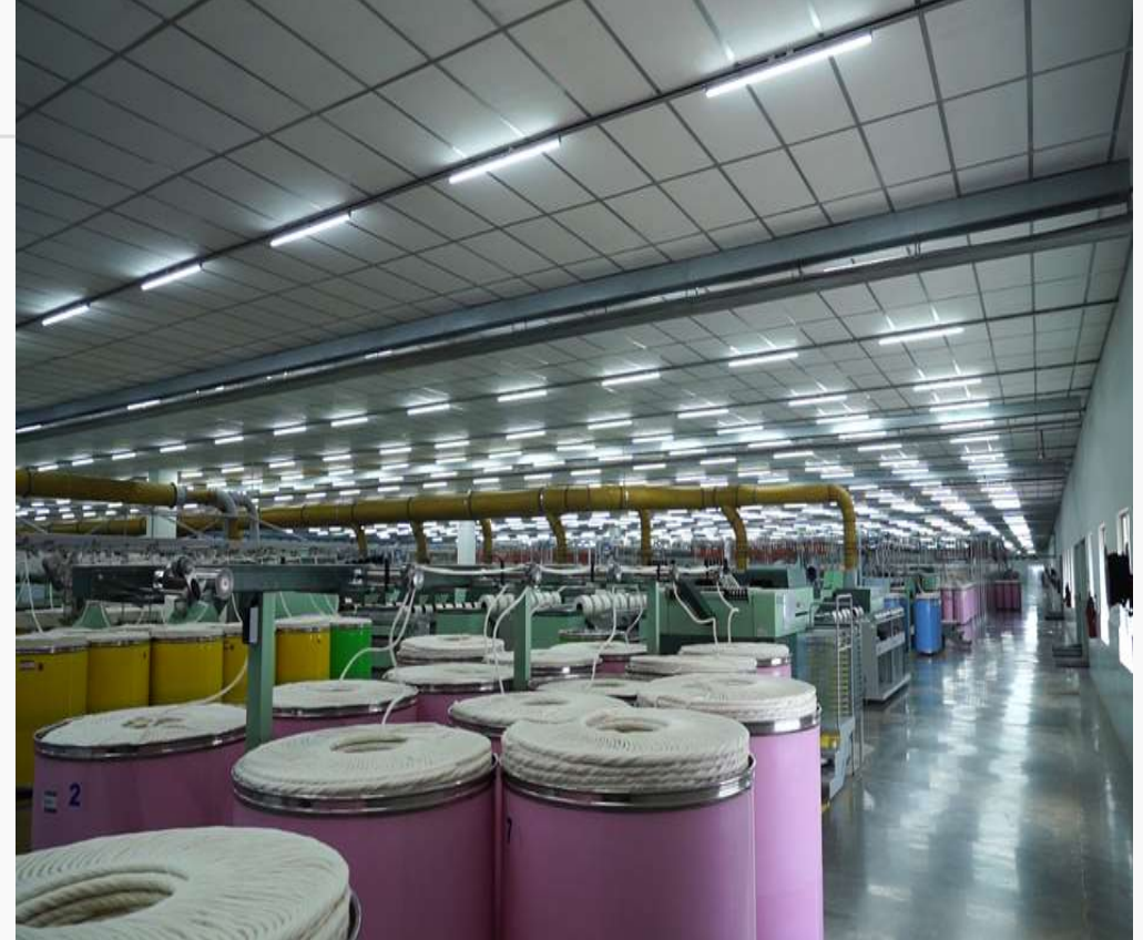
Electrification work of Spinning Mills
