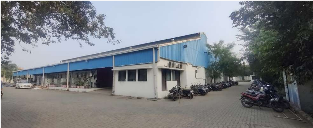
Location : XI-73, MIDC, HINGNA, INDUSTRIAL AREA, NAGPUR – 440 016 (M.S.) INDIA Area: 5,600 Sq. Mtrs. : Divisions Operated : Electrical Panels
