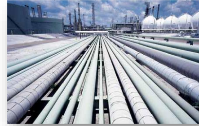
Anti Corrosive Material
