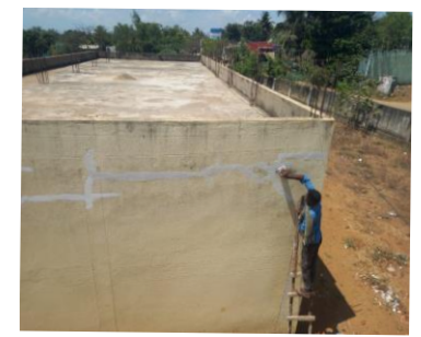
Repaired existing government run school building
