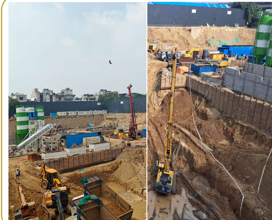
Excavation Work in Progress
