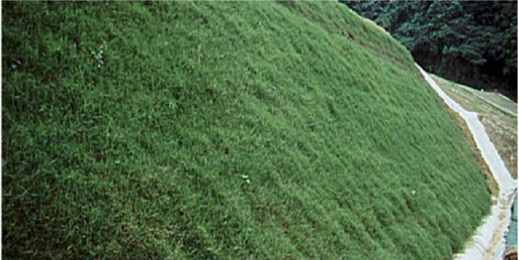
Slope Protection works for a project
