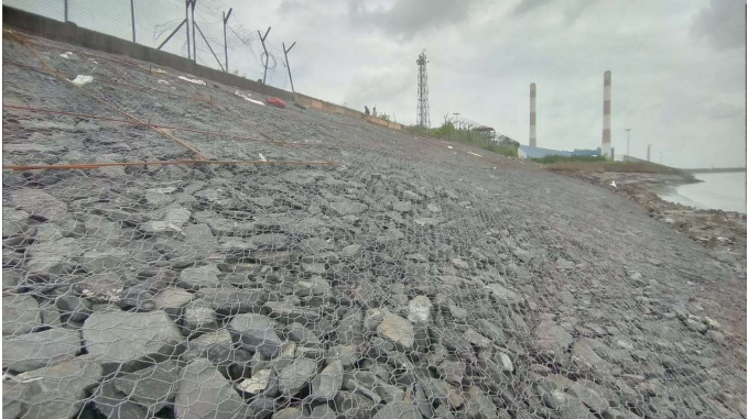
Coastal Protection works for a project in State of Gujarat
