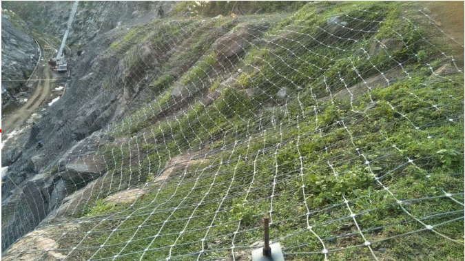
Rockfall Protection works for a project in state of Jharkand
