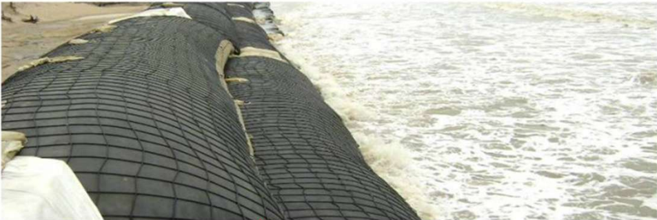
Coastal Protection works for a project
