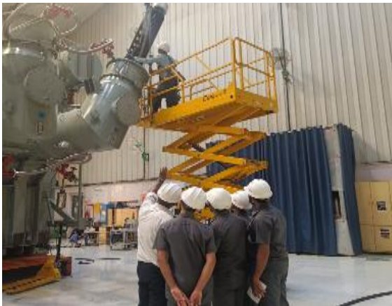
Working on mobile platform
