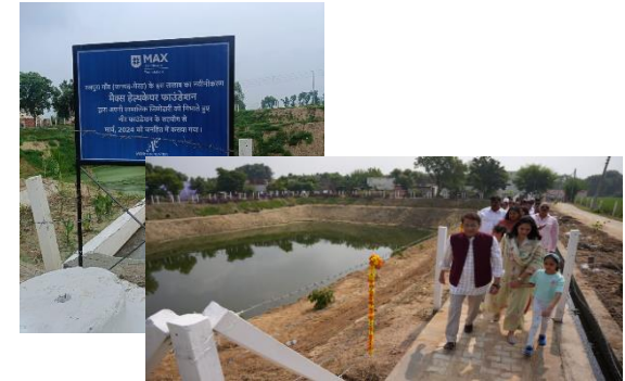
Construction of Pond in Meerut (Rajpura Village)
