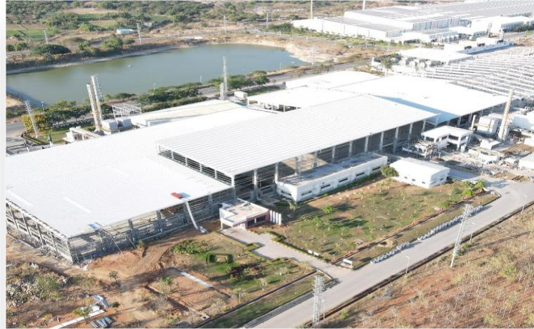
Tubular Battery Plant at ARGC – Chittoor
