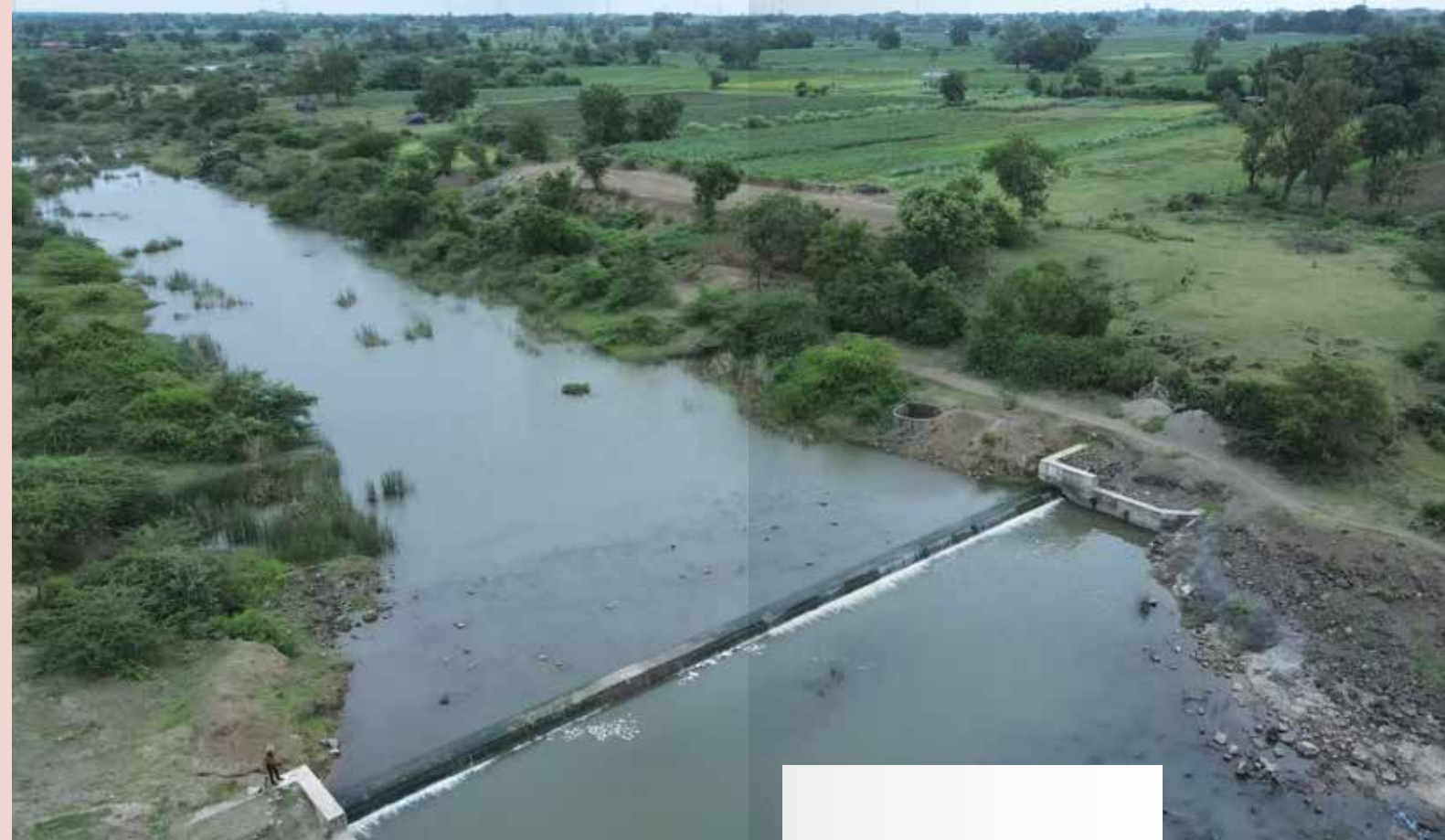
Zanjhmer check dam developed in collaboration with Narmada, Water Resources, Water Supply and Kalpsar Department of the Government of Gujarat
