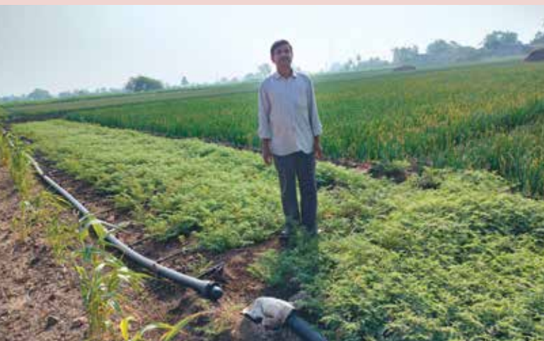
Drip Irrigation installation at farmer field
