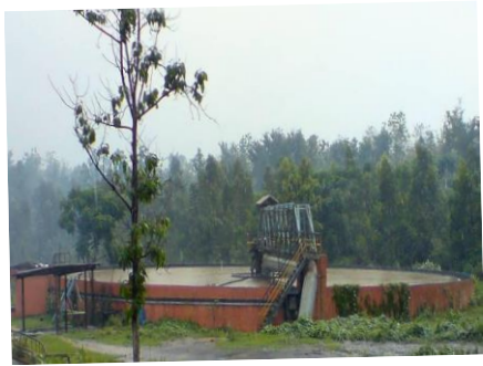
Primary Clarifier - Pulp
